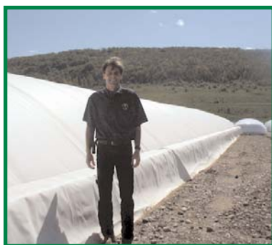
Anaerobic digester at a 750-head dairy farm in New York.
