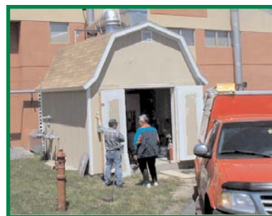
Microturbine shed, located at the Crouse Community Center.
